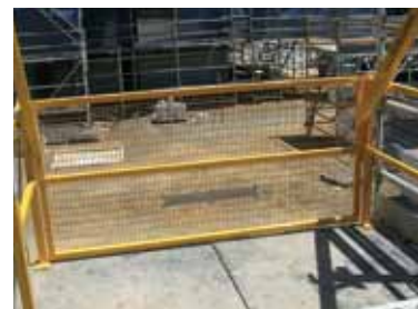
Watergate incorporated into scaffolding on a building site
